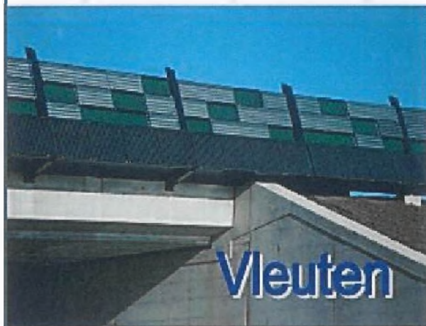
Sound absorbing noise barrier
