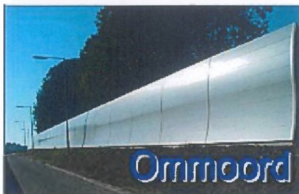
Sound reflecting noise barrier of aluminum
