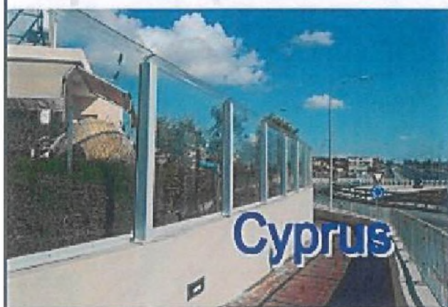
Sound reflecting noise barrier of acrylic plastic
