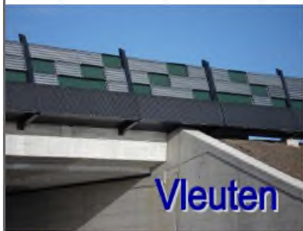
Sound absorbing noise barrier
