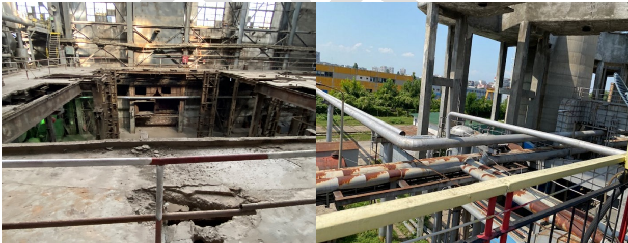
Figure 2-2 Site Visit Picture of Boiler Buildings and Piping
